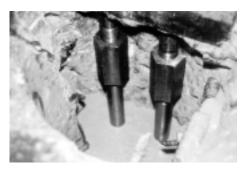
Fig. 4: An in-progress photograph of the replacement of dual anchor bolts after the first pour of epoxy grout. The isolation sleeving has not yet been installed.
