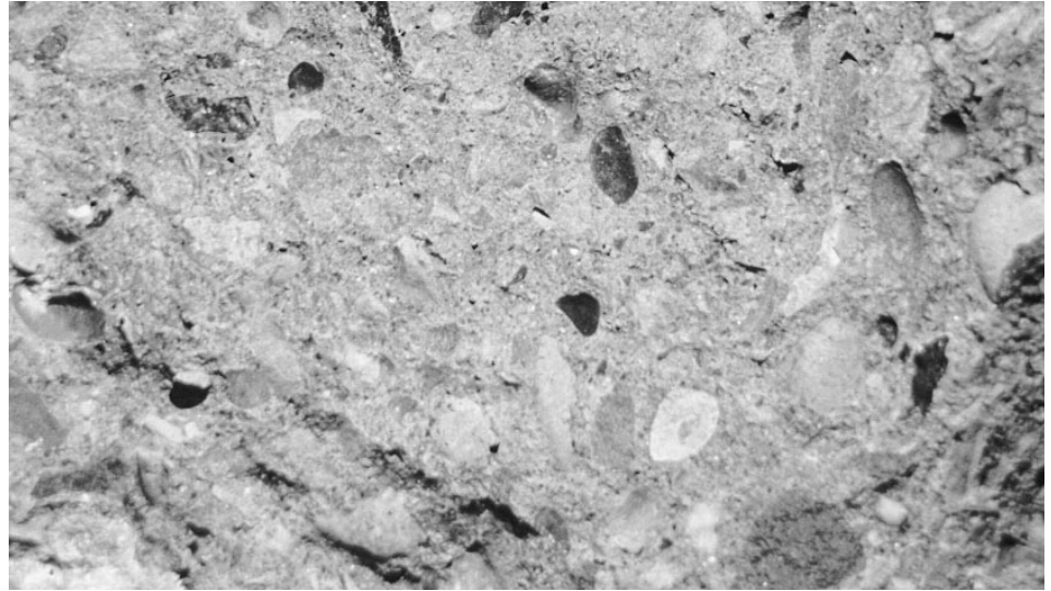
Figure 1: Proper chipping of the surface of concrete prior to grouting
