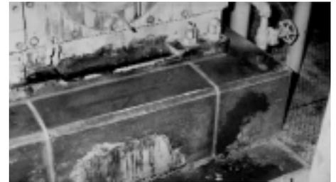
**Fig. 3:** A photograph after regrouting. Note the expansion joint at the anchor bolt and that the outer periphery of the machine base has been sealed with a fillet of silicone rubber.
