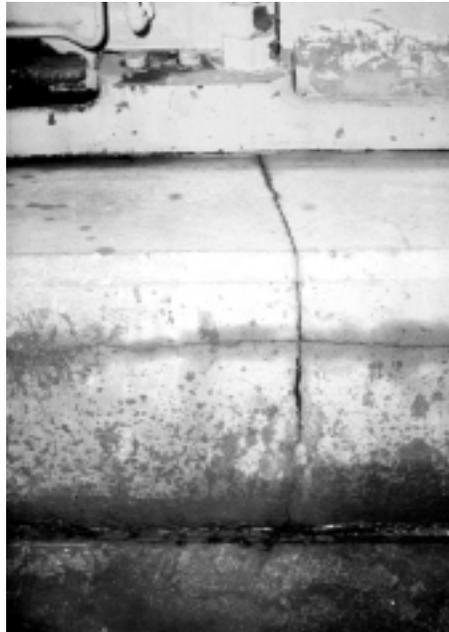
**Fig. 2:** A photograph showing foundation cracks at an anchor bolt. This crack is in a plane perpendicular to the crankshaft.
