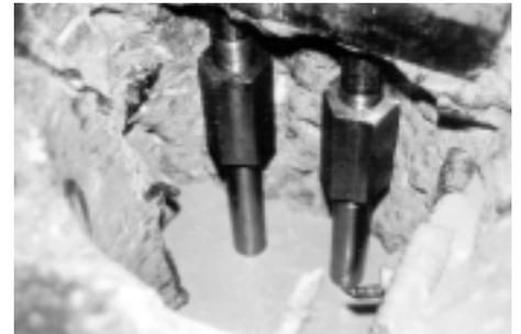
**Fig. 4:** An in-progress photograph of the replacement of dual anchor bolts after the first pour of epoxy grout. The isolation sleeving has not yet been installed.
