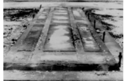
Fig. 2: This illustrates proper skid grouting.
