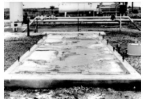
Fig. 3: Poor grout placement on a similar installation.
